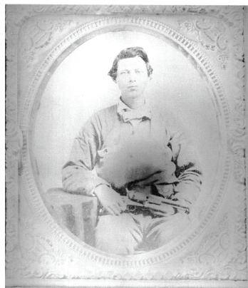
Wash. Achille Ferris, Company, H, 8th Texas Cavalry.
